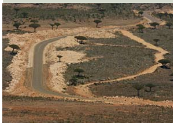
Figure 3. One of the badly landscaped roads on Socotra.
