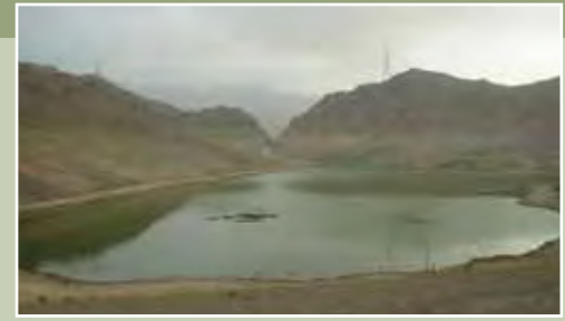
Fig 2. View of Ham Dam reservoir (© Christophe Tourenq).
