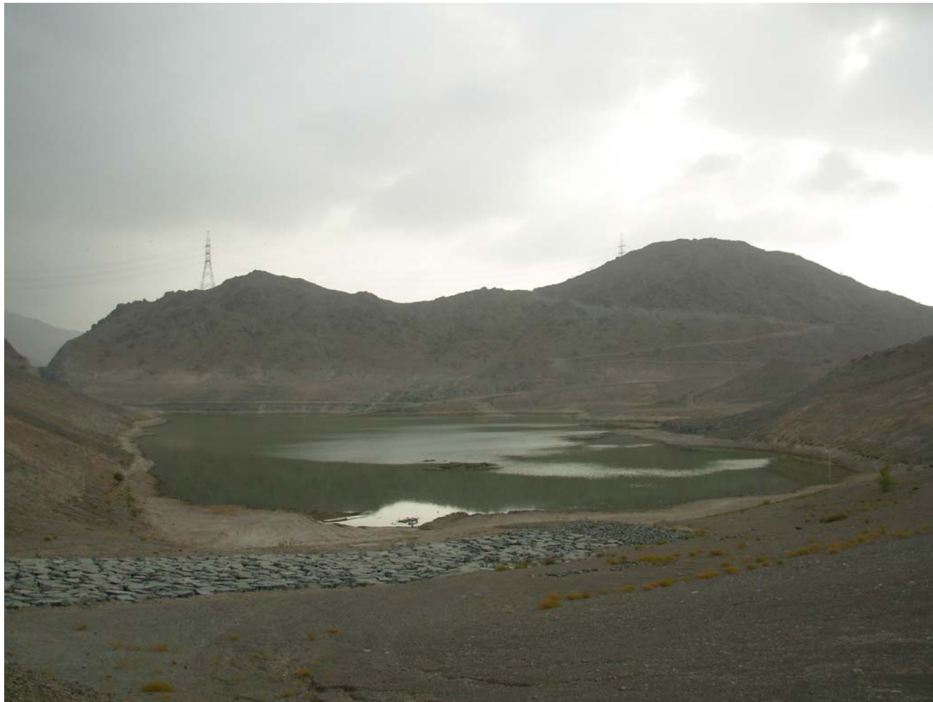
Figure 2. View of Ham dam D reservoir
